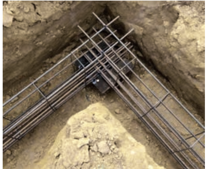
Cast-in-place beam
